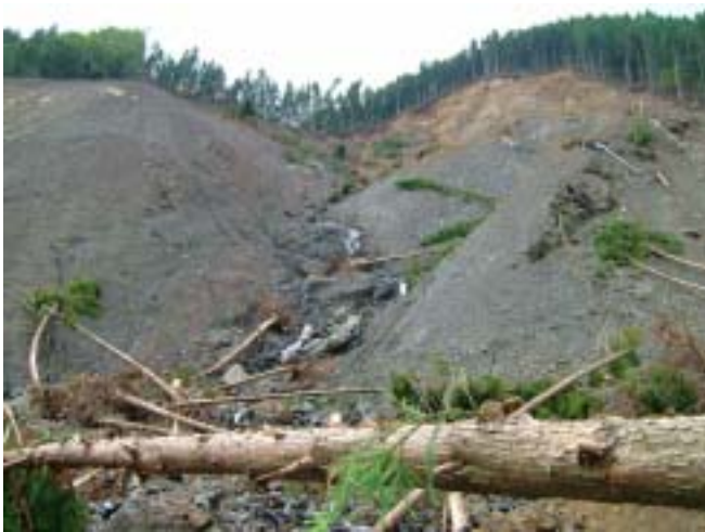
Photo 3 Kamagatani slope failure. Length: 220m, Width: 200m, Mean thickness of superficial fallen layer: ca.5m, Mean inclination: 31degrees, Volume of fallen soil mass:ca.1.3×10 5 m 3 . Small torrent in the center of slope and spring point in the mid slope where the boundary of bed rock (weathered crashed muddy rock) and superficial thick layer
